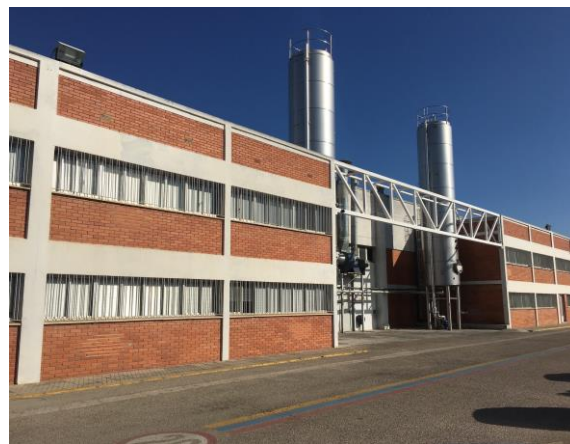
SOR offices, before renewal
