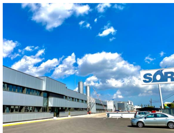
SOR offices, after renewal
